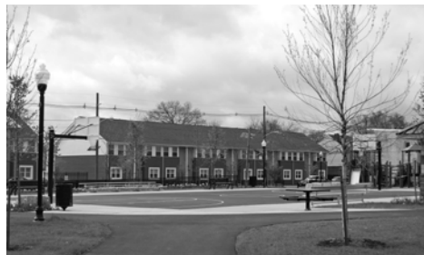
Homes built by BCHT in 2012 win 2015 Phoenix Award for exemplary brownfield revitalization
